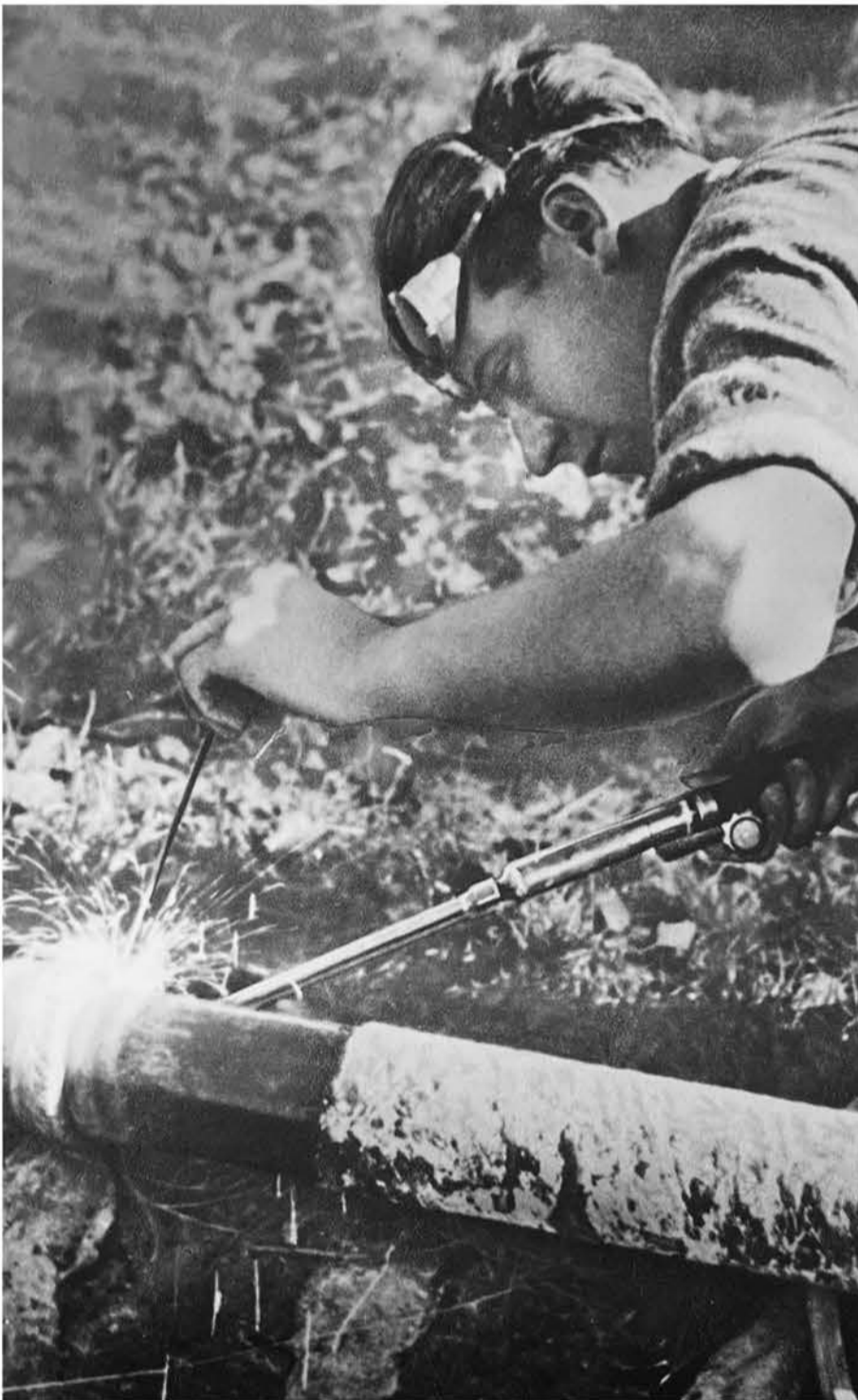
Laying of pipes in the Yvelines
